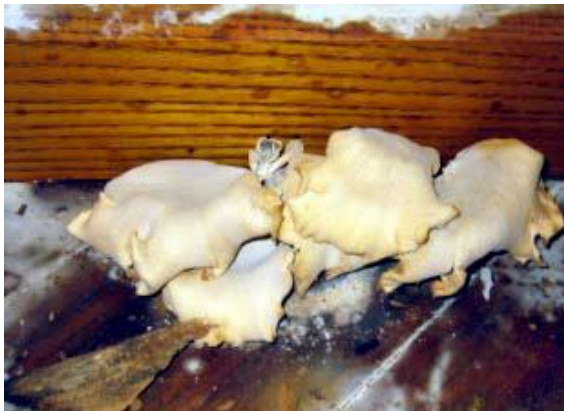
Mushrooms produced on hardwood floor where there has been long-term water incursion. (Unknown or anonymous author. Image courtesy of Dr. Chin S. Yang Guidance for Clinicians on the Recognition and Management of Health Effects Related to Mold Exposure and Moisture Indoors Page 15)
