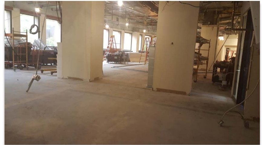
Academic Building Renovation: Demolition Complete in New Wellness Center Space
