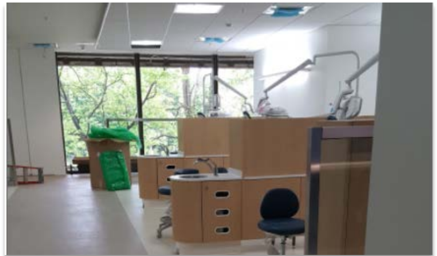
Clinic Building Renovation: Dental Clinic on 1 North Nearing Completion
